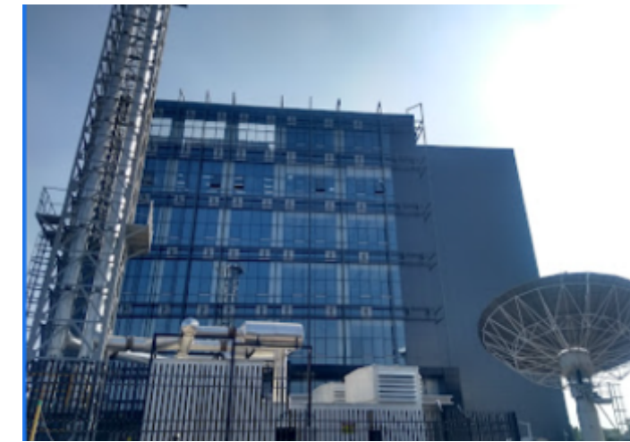
STTG Data Centre, Chennai & Pune
