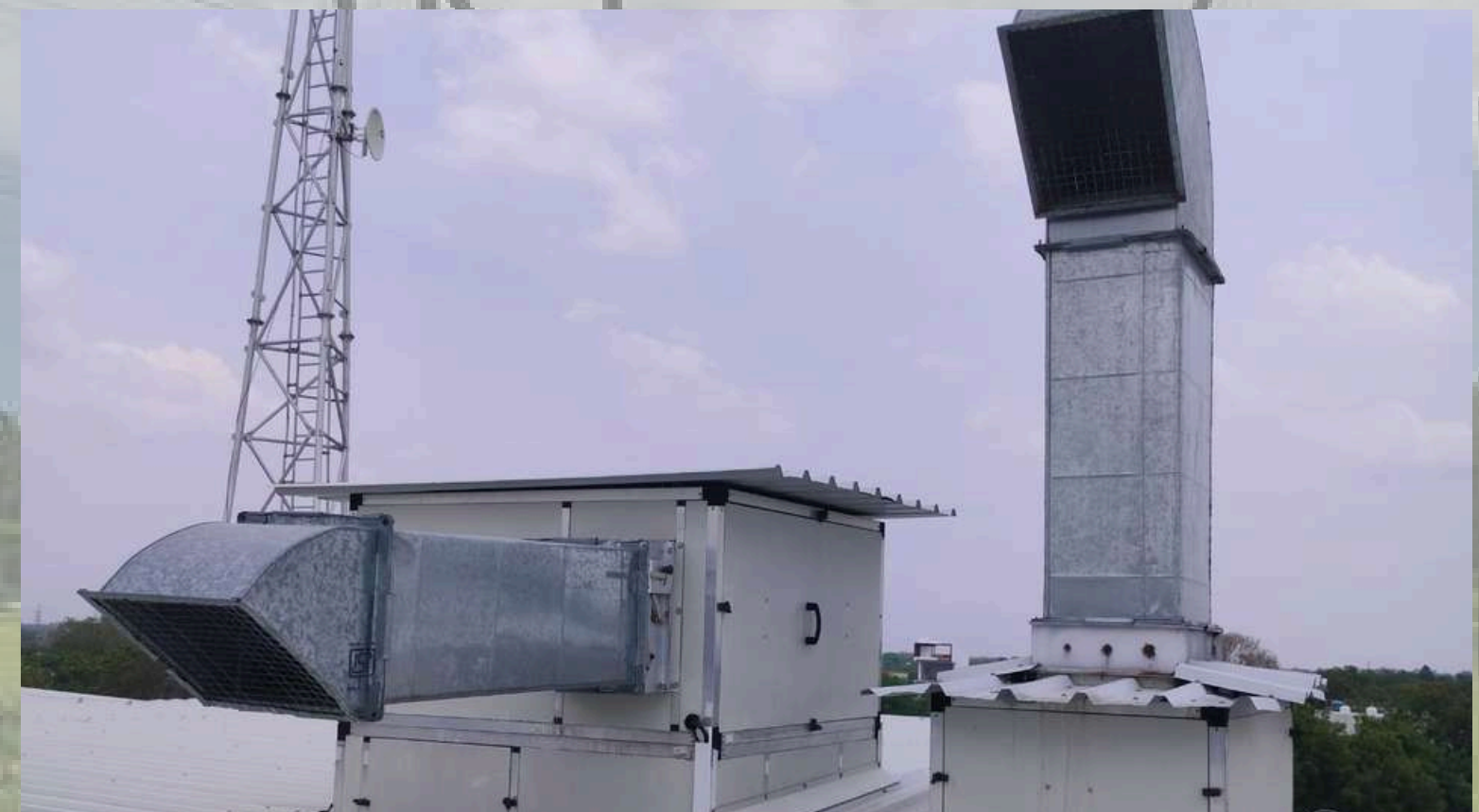
Evaporative Cooling System
